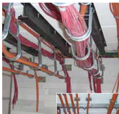
Installation within fire chamber.
